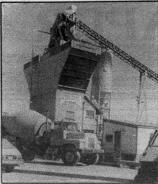
RULED OUT — Sebastopol Ready Mix won't be washing gravel in nearby Laguna. THE PAPER/Mazzullo
